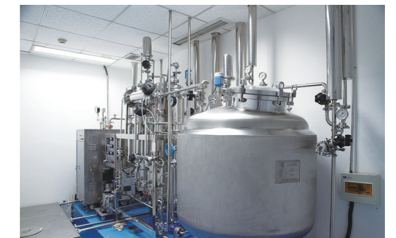
Distilled water system to ensure endotoxin below 0.015 EU/ml
